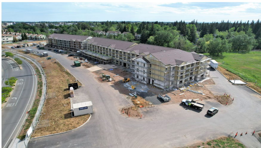
Photo courtesy of Sunseri Construction
